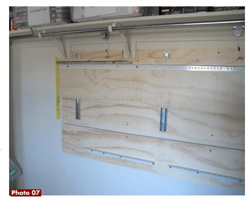
**Photo 07.** You should then be able to insert the traveler with its sliding rails now on the back of the traveler into the wall mounted rails and move the traveler up and down with no binding. This will be too heavy to stay up by itself, so make sure you still have those 2X4s(not pictured) around to support the traveler while you finish up. You will now need to counterweight the traveler.
